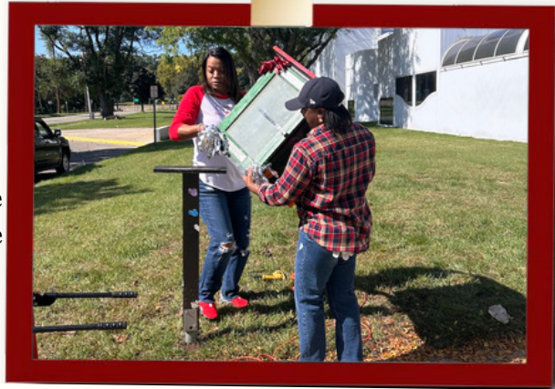
Soror Ta'Alea Fluellen helping Ms. Deanna Roberts repair the library mailbox and put back in place
